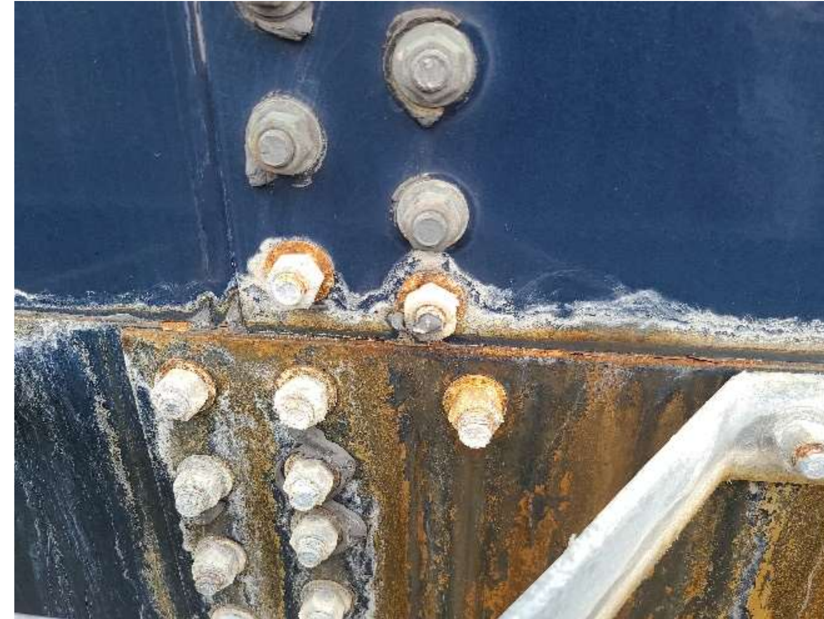
Exterior Bolt Corrosion and Leak
