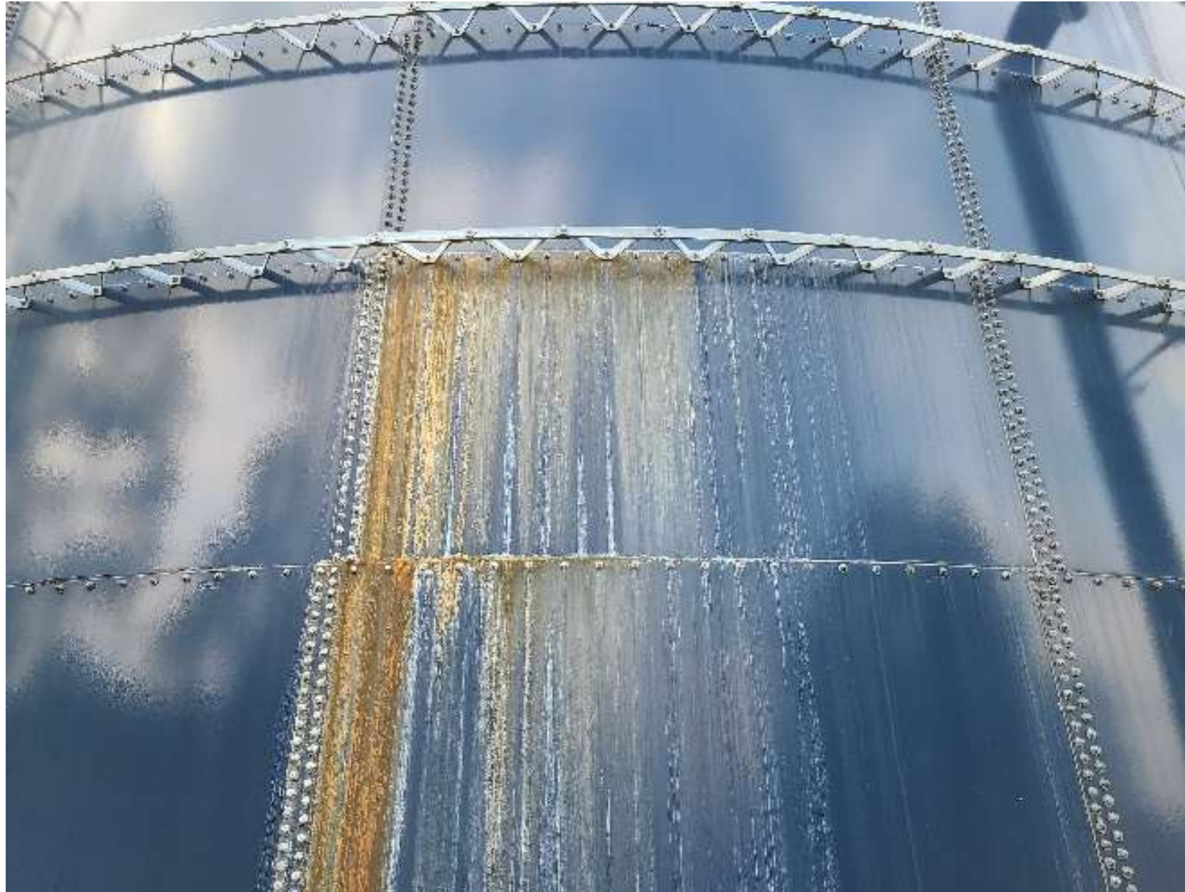
Exterior Leak and Deterioration
