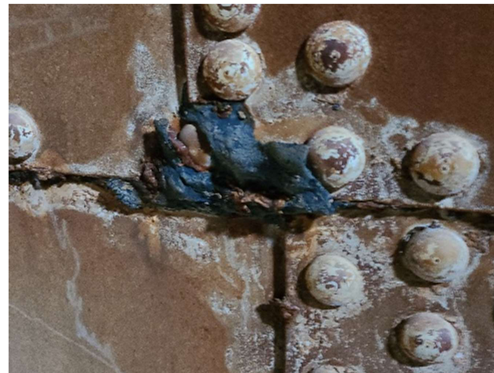
Interior Sealant Deterioration
