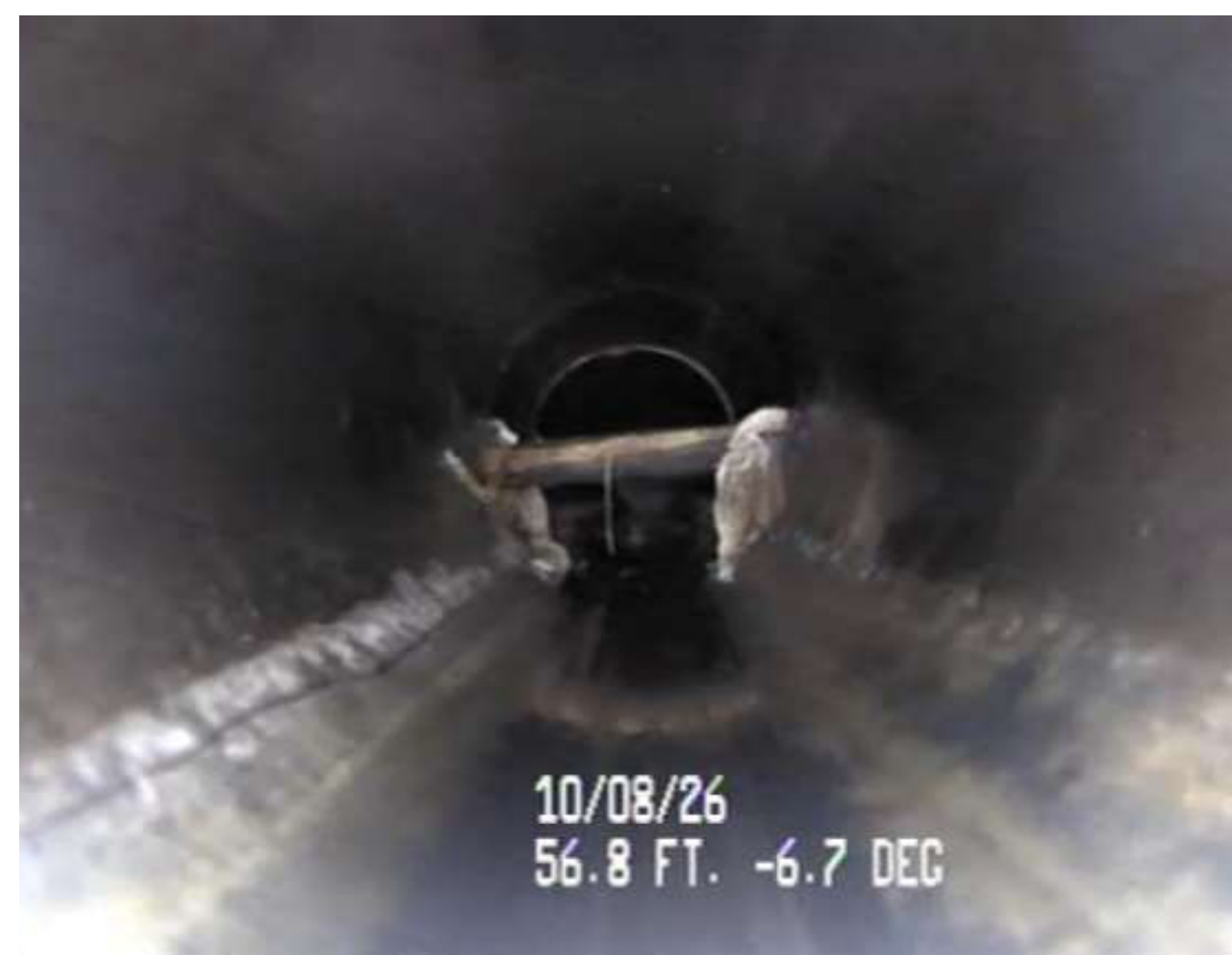
Pipe Blockage Between MH 104-141
