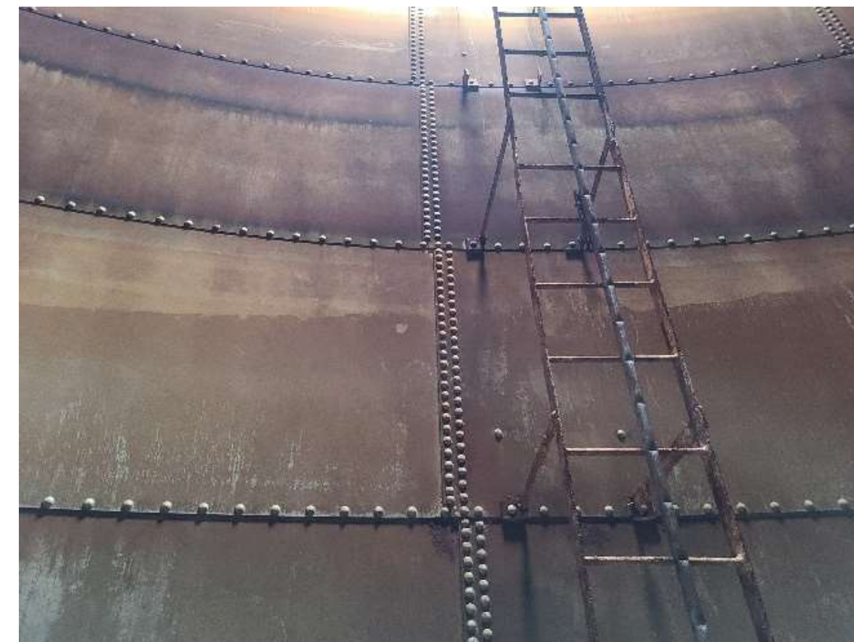
Ladder Corrosion
