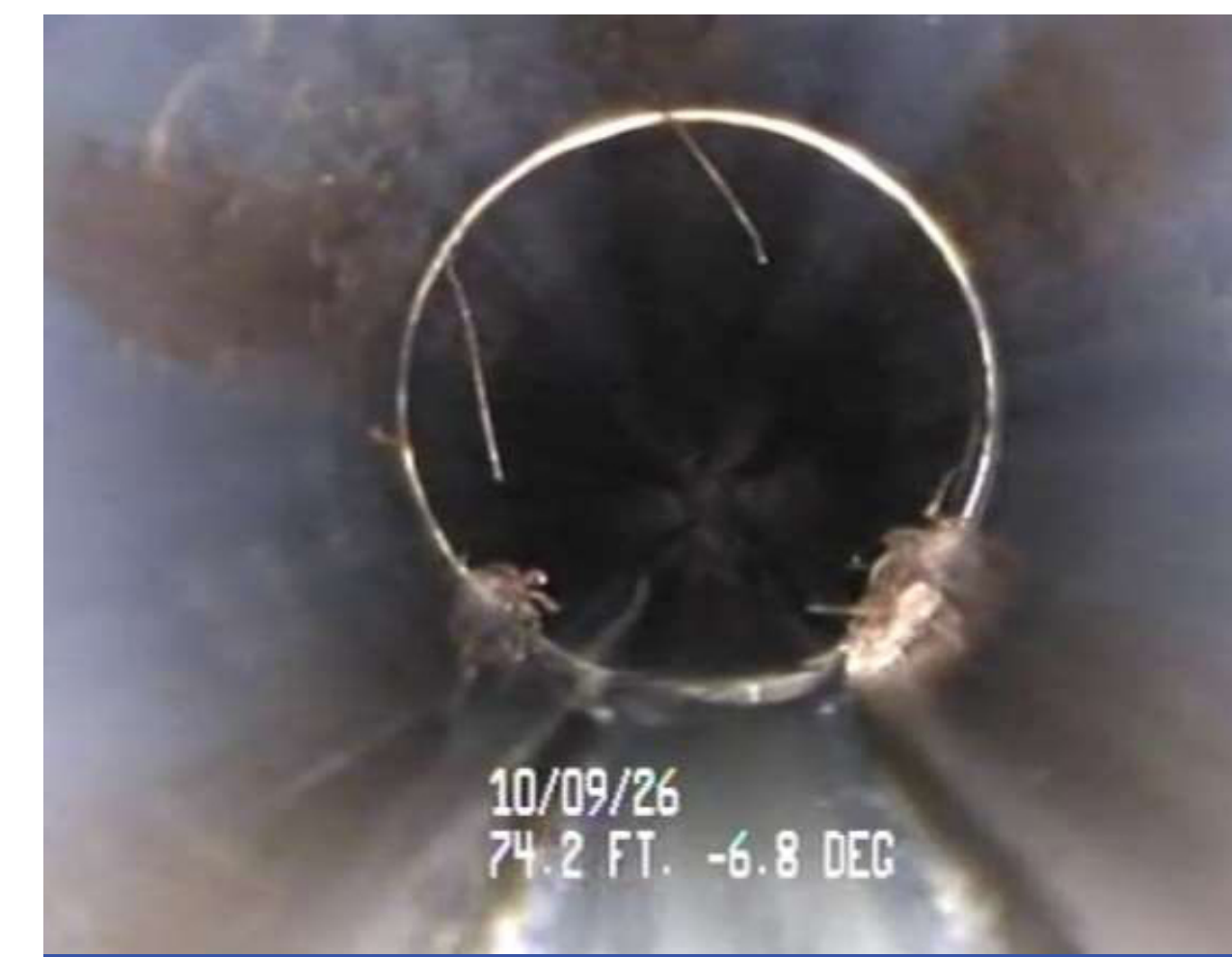
Existing Root Joint Between MH 127-128
