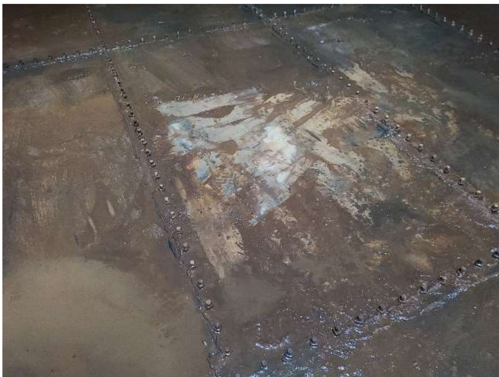
Interior Floor Deterioration
