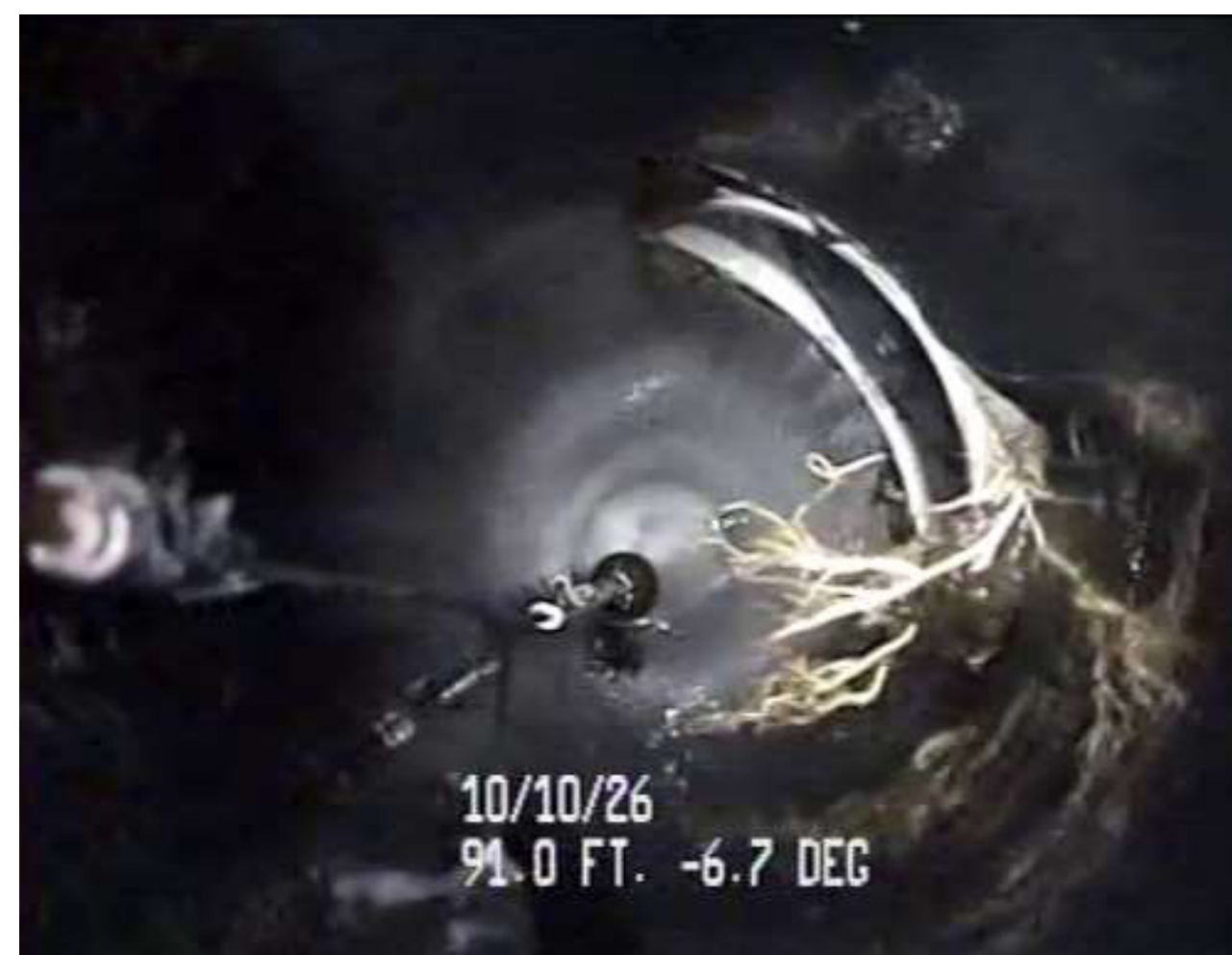
Existing Pipe Crack and Root Between MH 90-92
