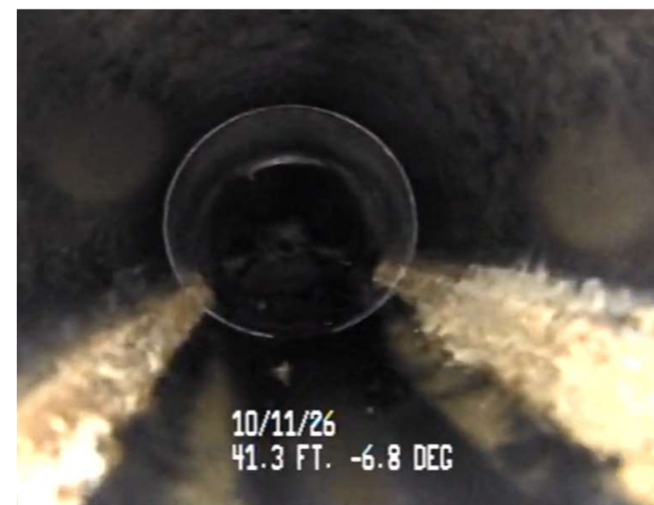
Existing Pipe with Grease Between MH 119-120
